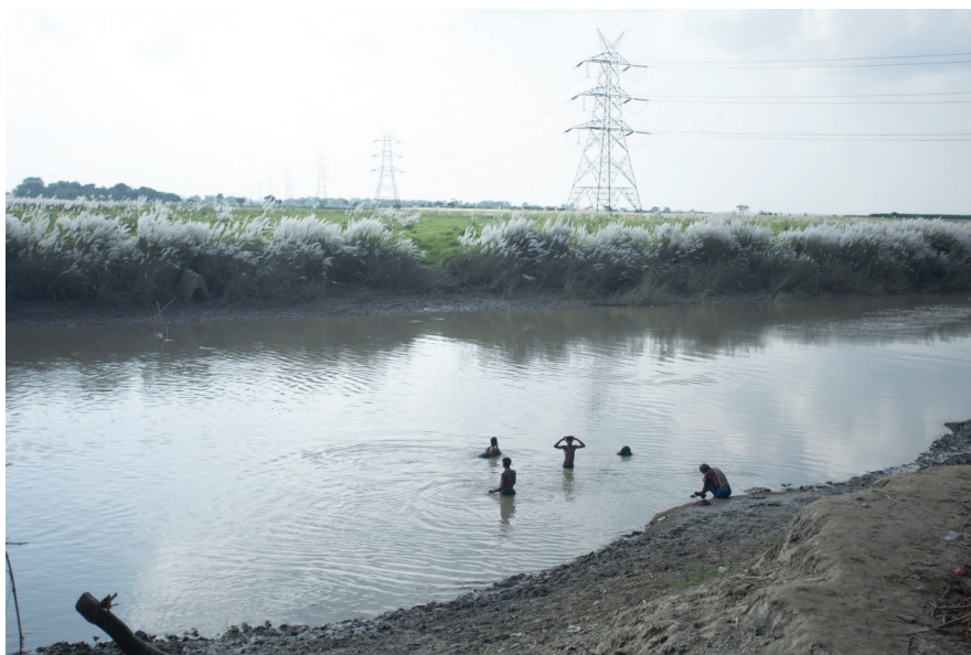
Figure 12: Power line from India entering Bangladesh through Ramkrishnapur (Source: IRADe)
